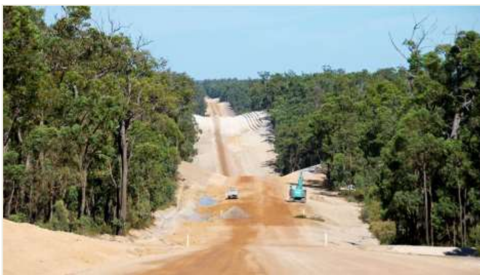
Mowen Road construction project
