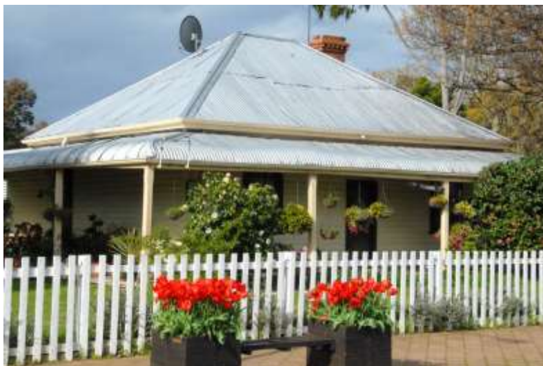
Character residence in the Nannup townsite
