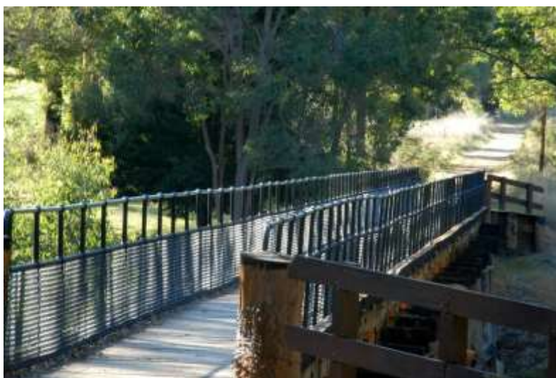
Old Railway Bridge over the Blackwood River
