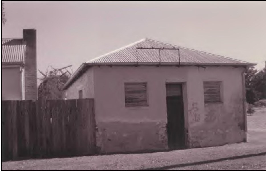
Photo Dated: Dec 1994 WESTPAC BANK BUILDING WAREHOUSE
