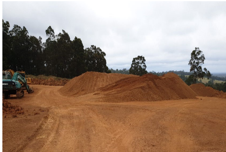
Fig 5: Completed Stage 1 area, now used as a stockpile and processing area, can serve as a refuge.
