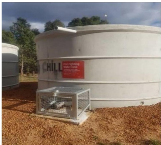
Strategic 47,000 Litre Concrete Tank & Protected Fittings
