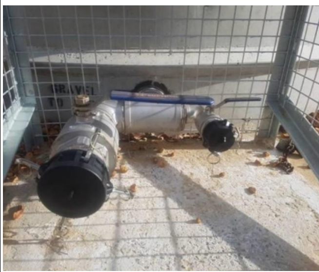
Strategic 47,000 Litre Concrete Tank & Protected Fittings
