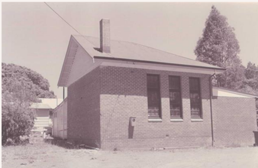
Photo of the "Old Kindy Building" (or "Nannup Pre-Primary Centre") (Source: inHerit, Heritage Council)
