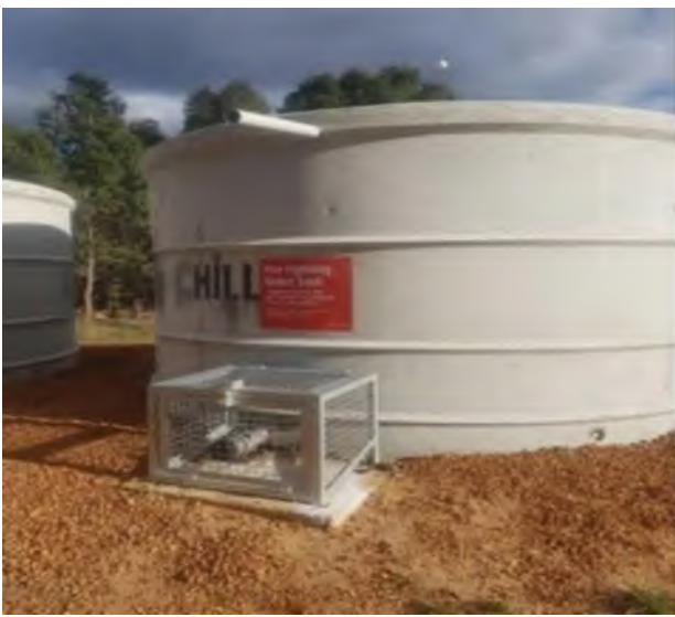
Strategic 47,000 Litre Concrete Tank & Protected Fittings
