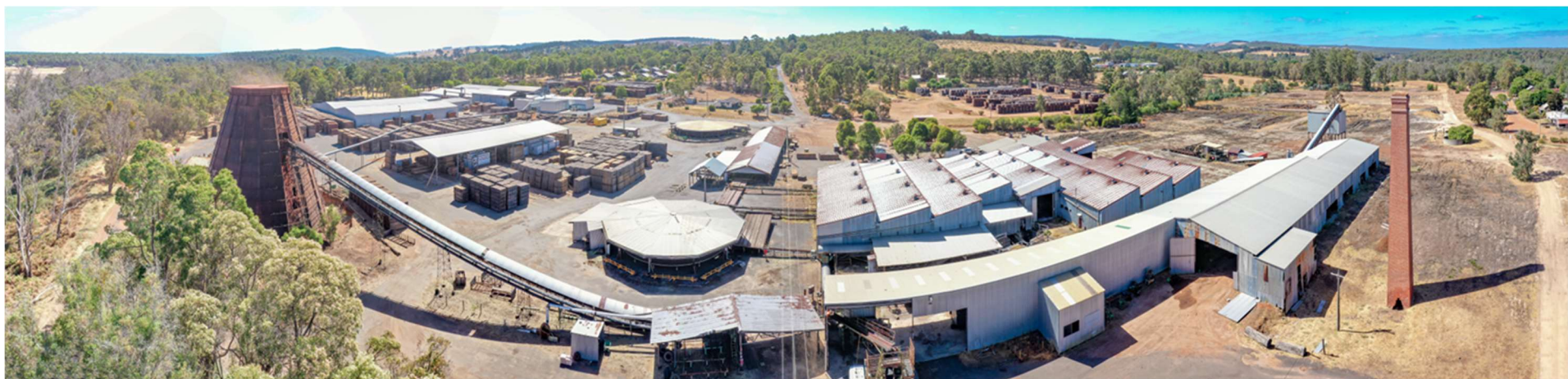
Figure 21: Panorama of the core Mill site and operational buildings – Looking east over the site operations
