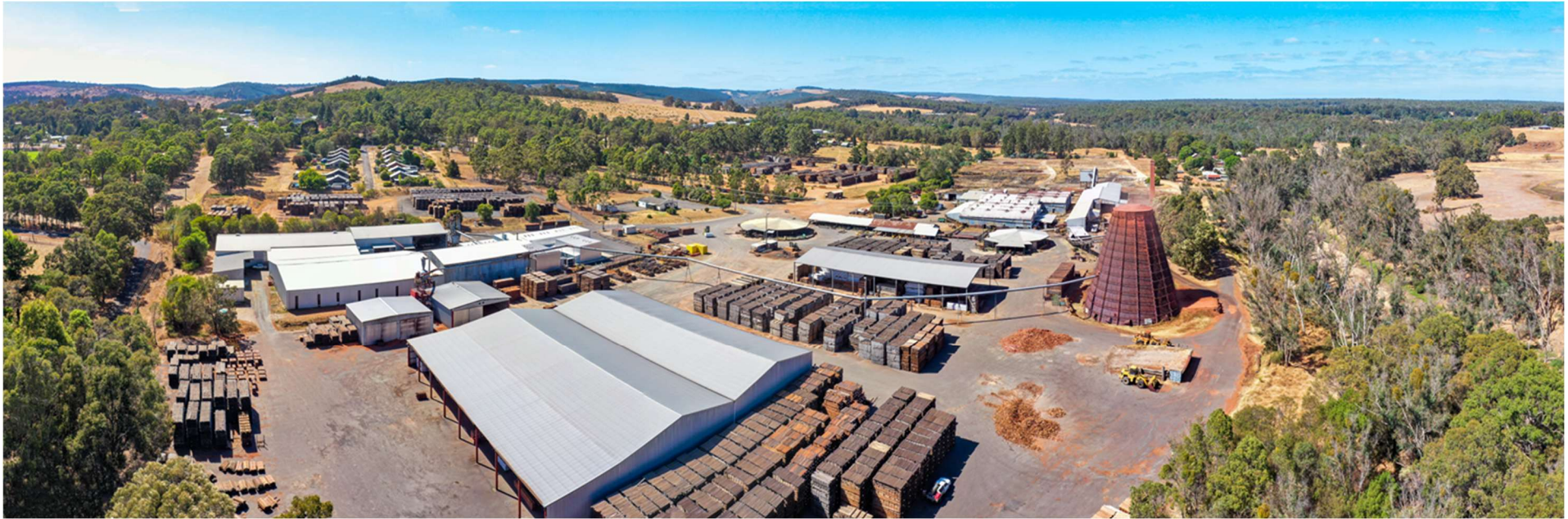
Figure 19: Panorama of the core Mill site and operational buildings – looking south over the site operations
