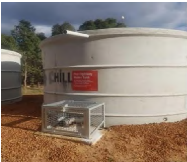
Strategic 47,000 Litre Concrete Tank & Protected Fittings
