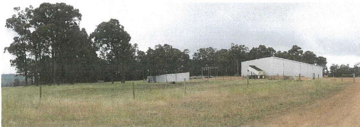
Fig 6: The main shed.
