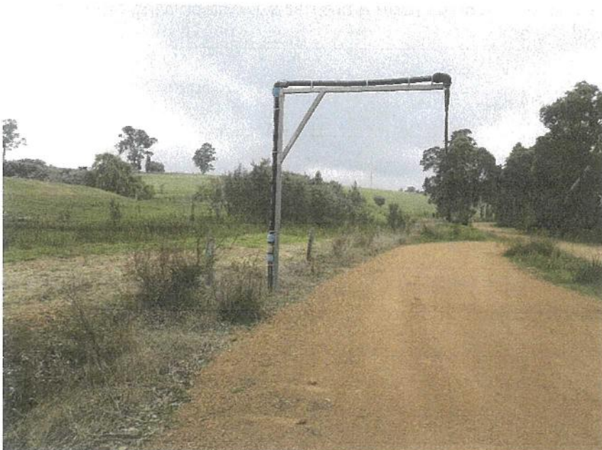
Fig. 8: Gravity fed standpipe off Mount Leewin Loop Road.
