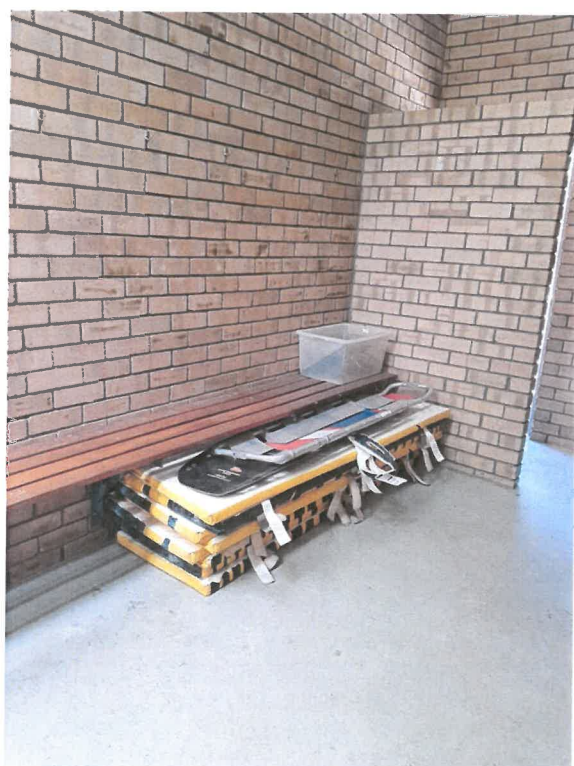
Existing change rooms
