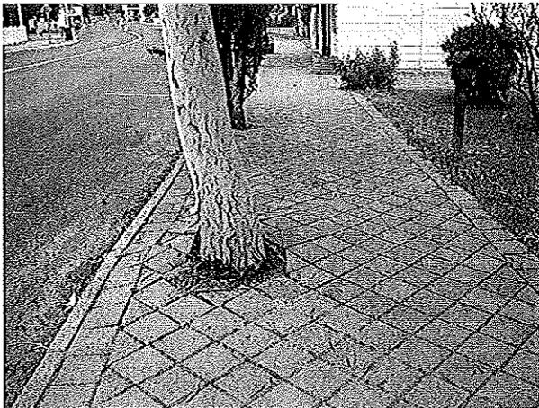
Brick paving footpaths are uneven as a result of tree root damage.
