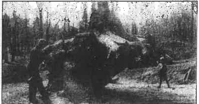
Johann removing tree trunk with hand pick from 'Pondulla' homestead site 1928 with son Robert watching.
