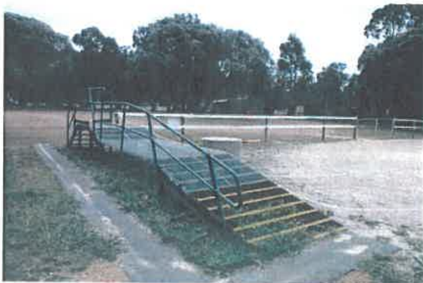
Photo: Mounting ramp
